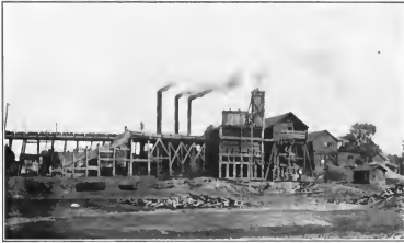
TIPPLE AND POWER HOUSE, CENTRAL MINE, CENTRAL CITY
